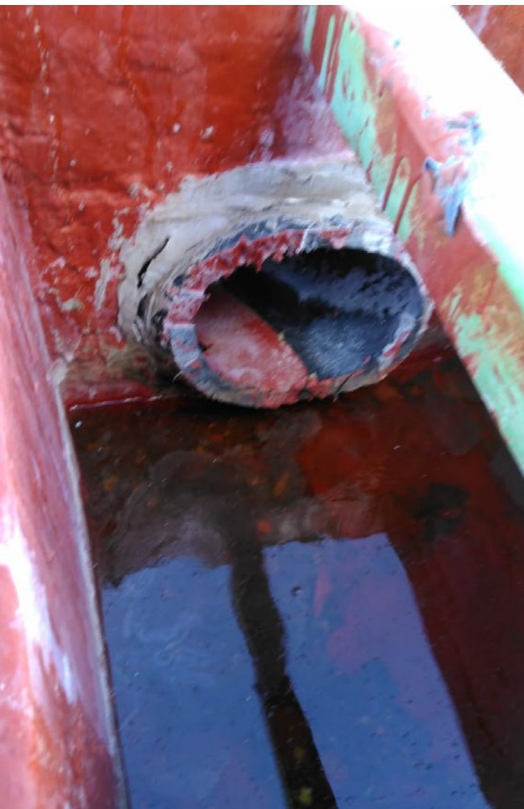
Unloading Platform and First Chamber
