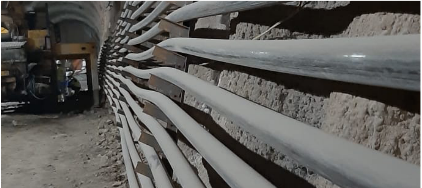
Installation of Pexgol pipe to transport fiber optic cables.
