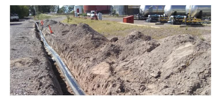
Installation of a fire supply network in a oil treatment plant.
