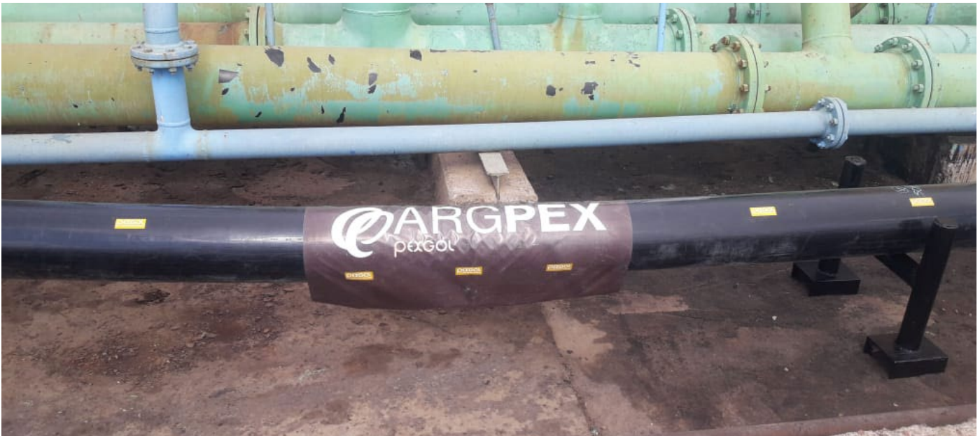
Installation of Pexgol pipe in a formation water treatment plant.
