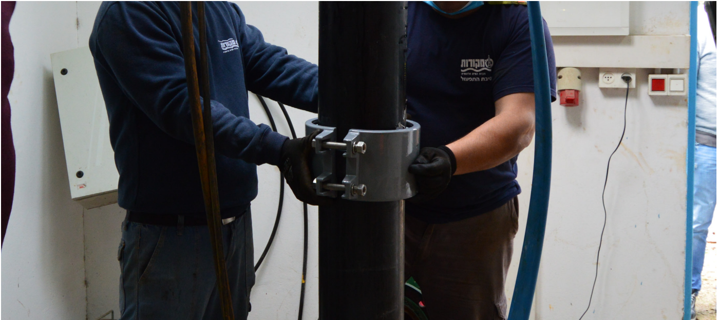
Installation of a borehole with pipe in sections for reduced space.
