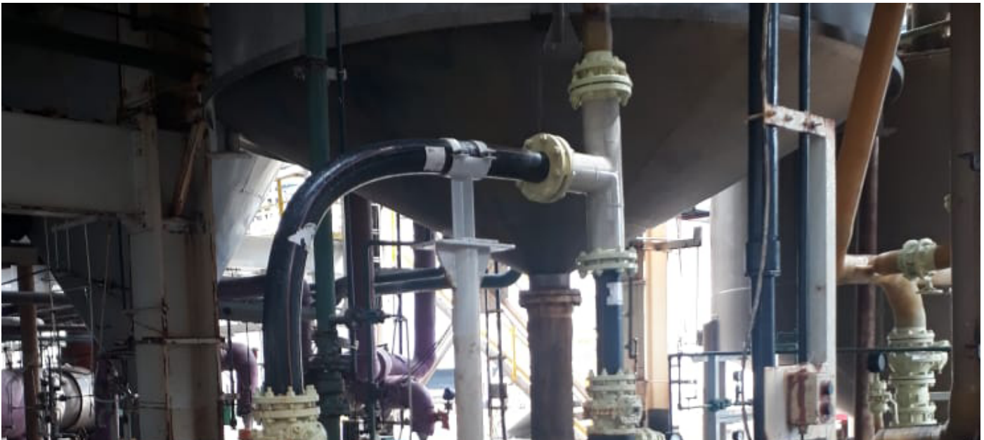
Pexgol fittings for brine transportation at a Brazilian chemical company.
