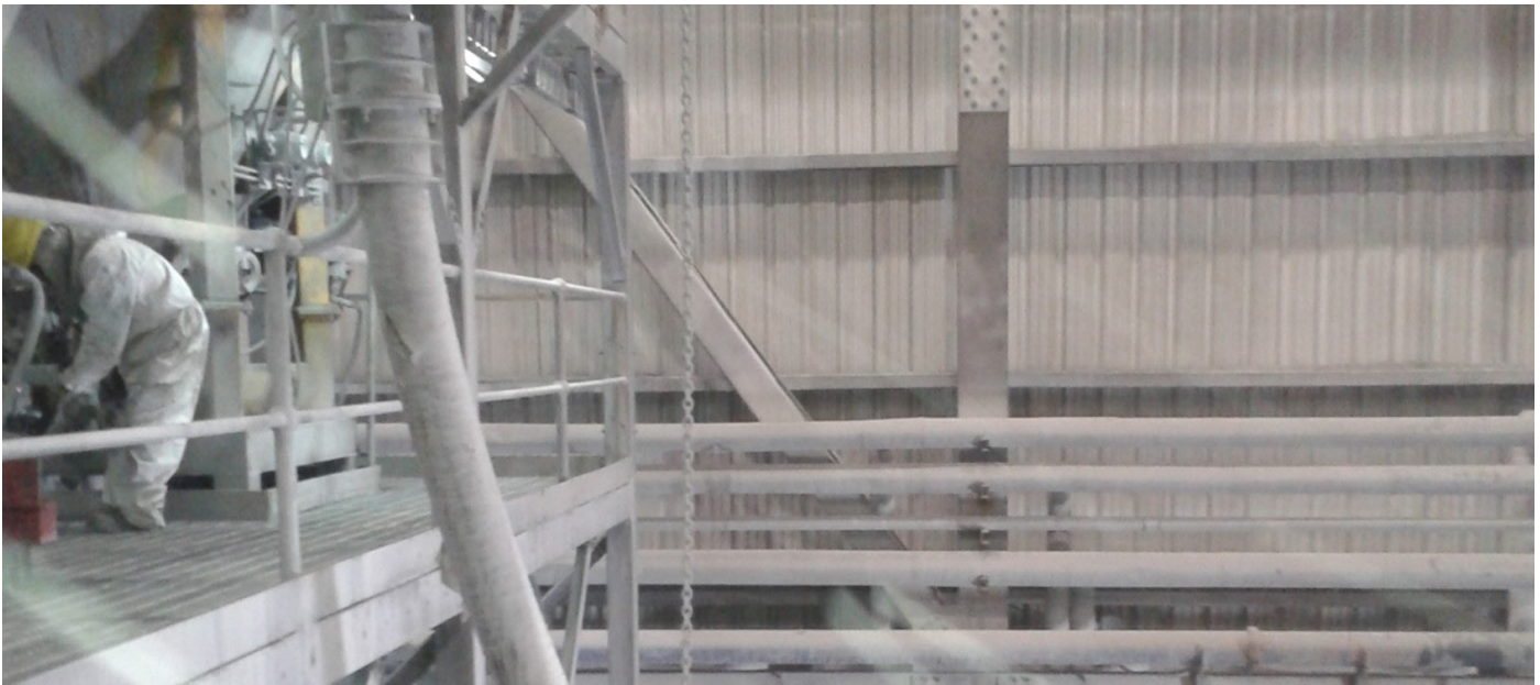
Installation of Pexgol pipe for the transport of abrasive tailings.
