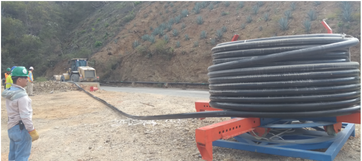
Installation of Pexgol pipe for transportation of mining tailings.
