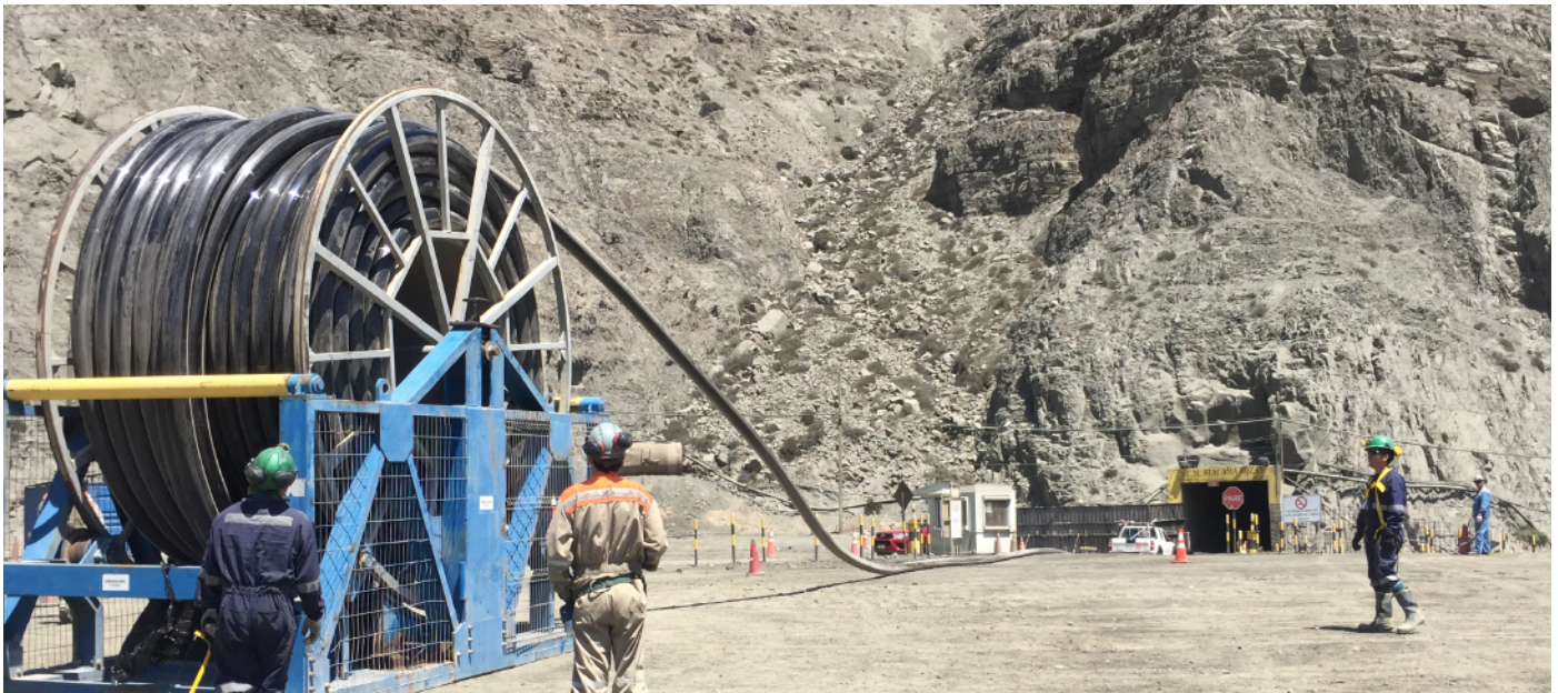
Replacement of a drainage line in an underground mine.
