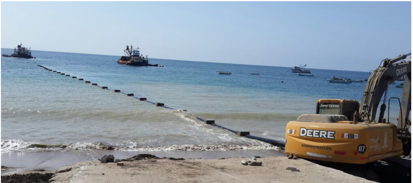
Installation of Pexgol pipes to transport fish.
