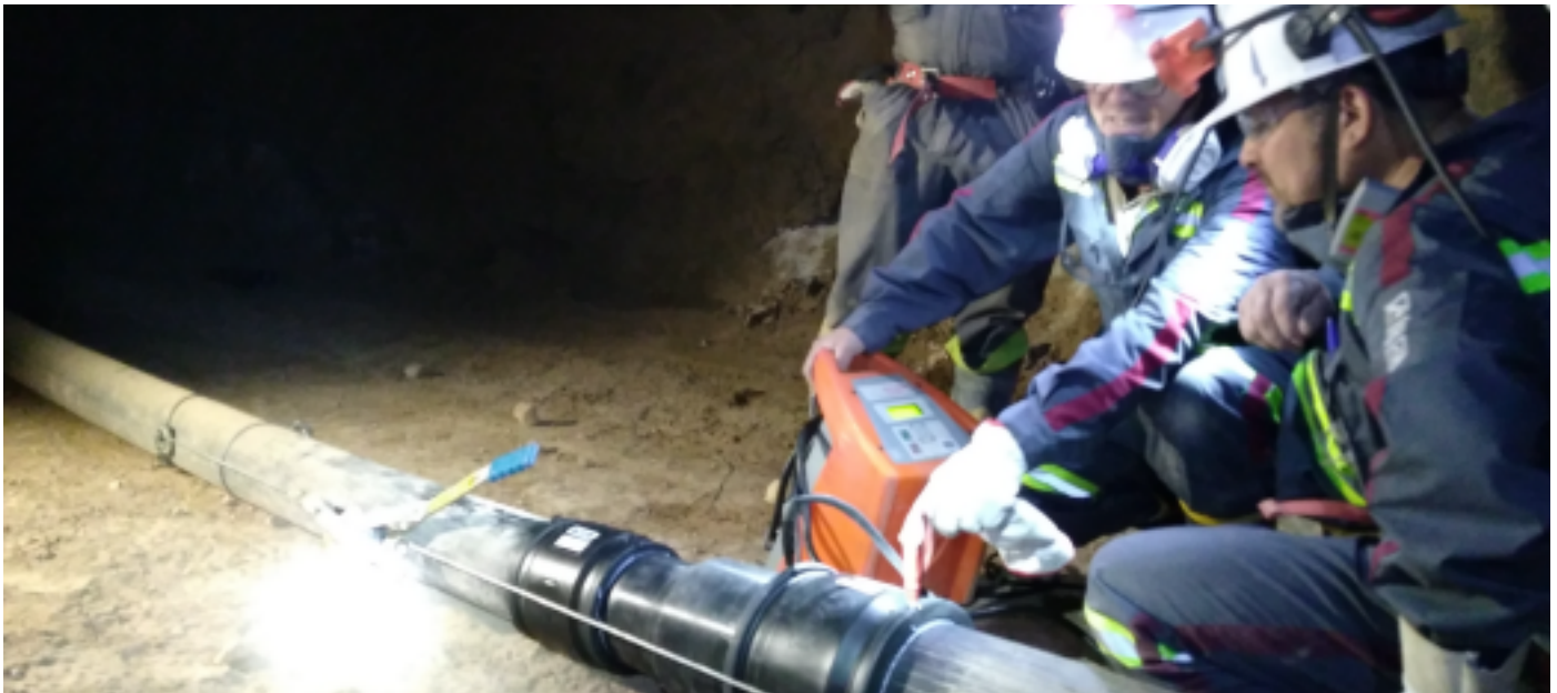
Installation of Pexgol pipes for drainage of an underground mine
