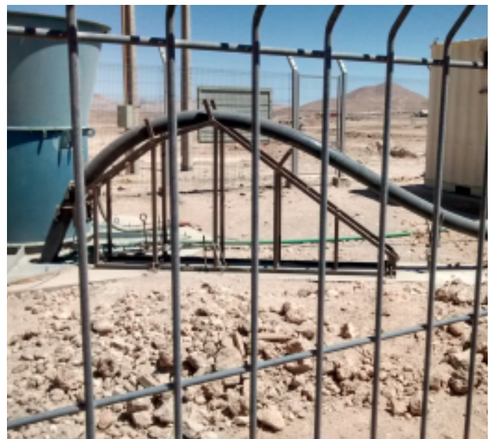
Ventilation chimney entry
