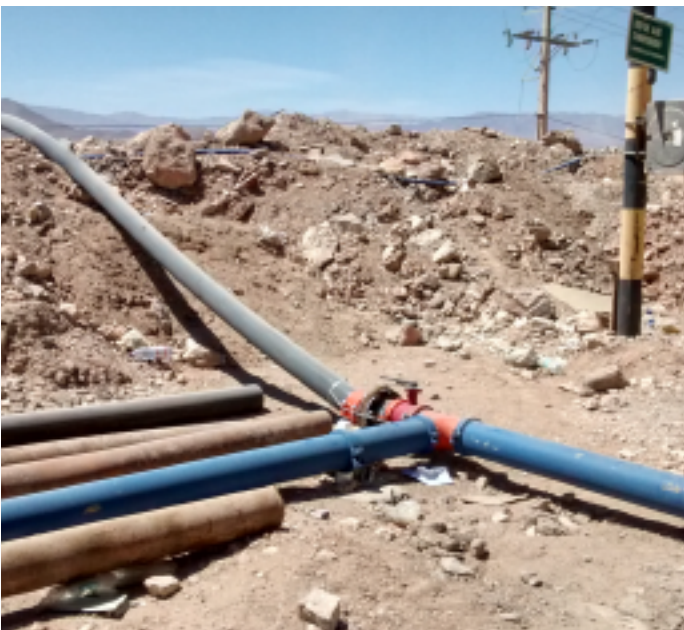
Compressor output connection
