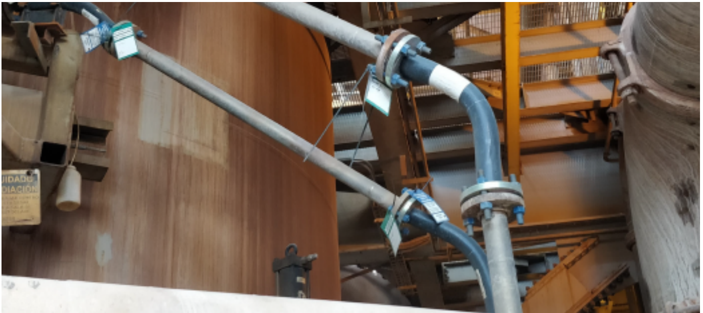
Replacement of titanium pipes by Pexgol pipes to transport acid solution.
