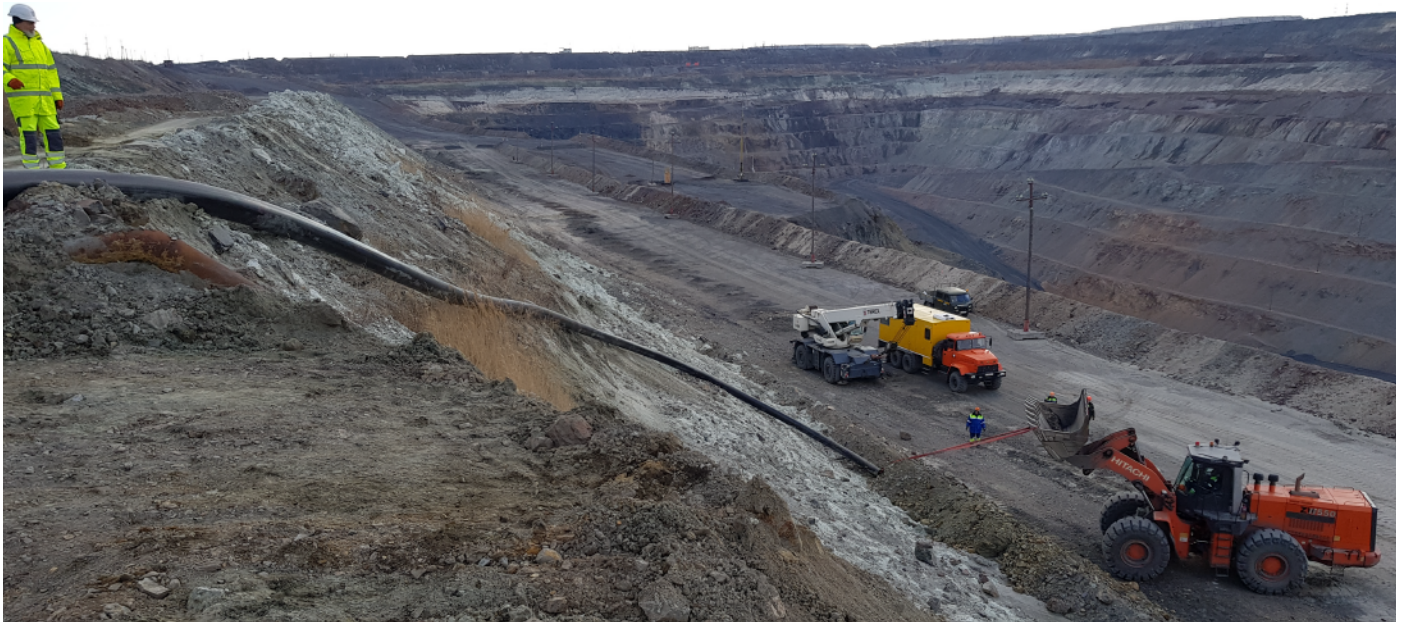
Vertical mobile Pexgol installation on the rocks for mine dewatering.
