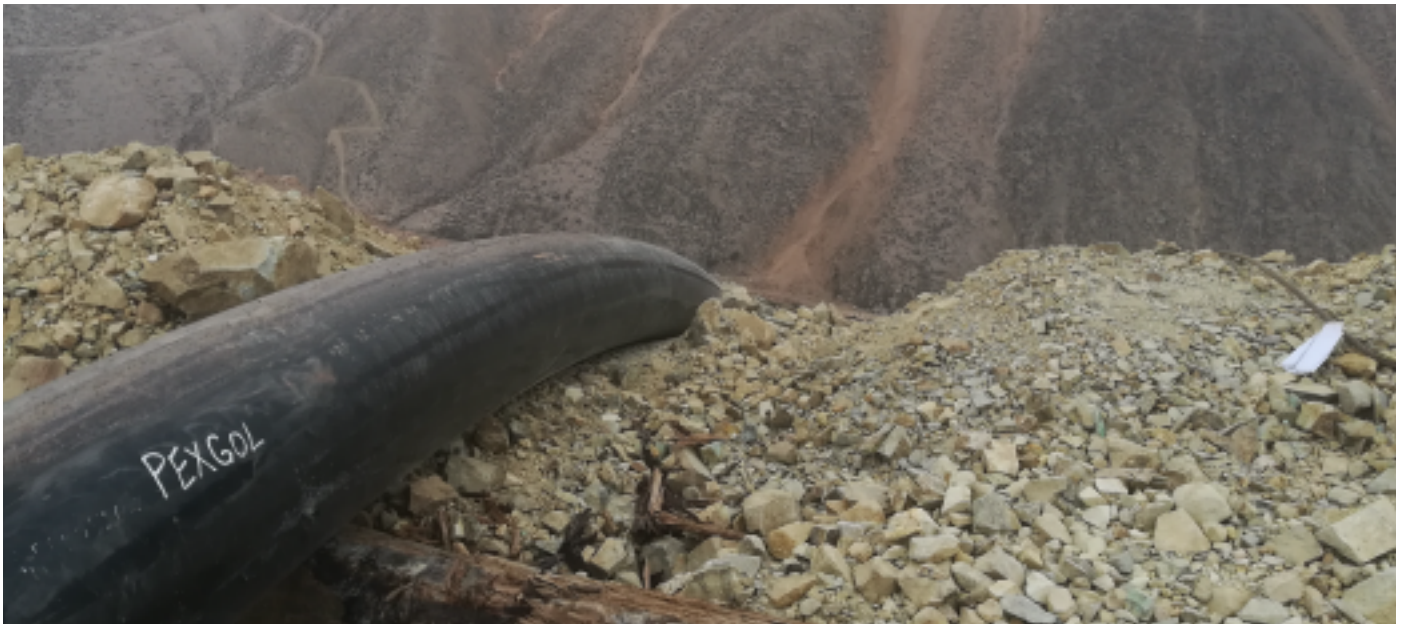
Transportation of river water in rough terrain.
