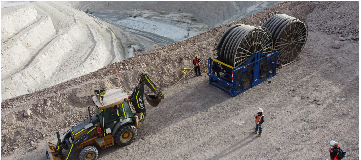
Pexgol pipe installation for open pit mine drainage.
