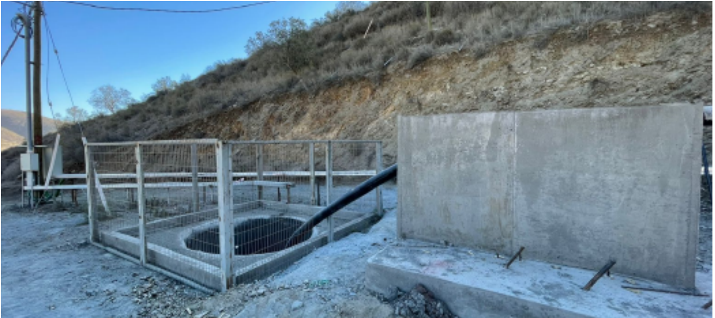
Installation of Pexgol pipes through a chimney for compressed air.
