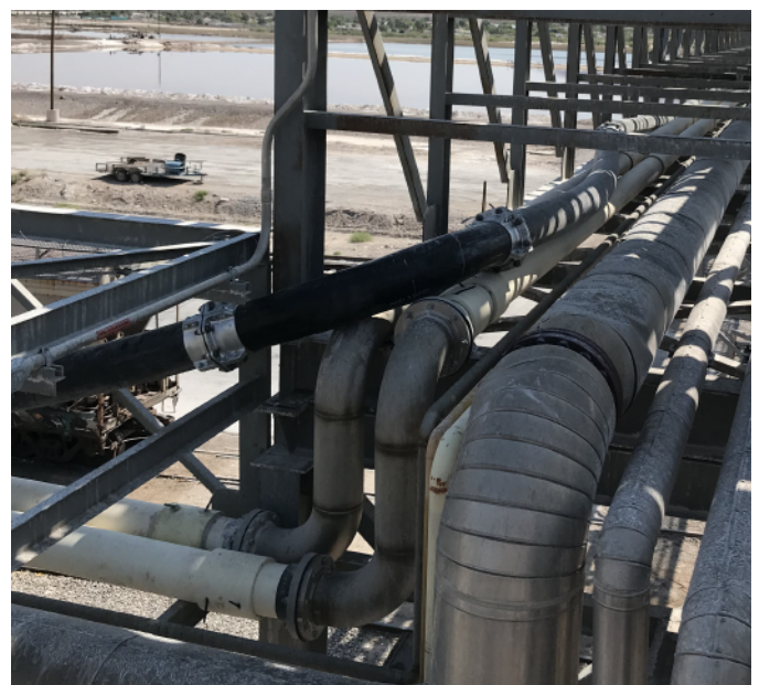
Thanks to the flexibility of the Pexgol pipes in many sections, prefabricated elbows were avoided.
