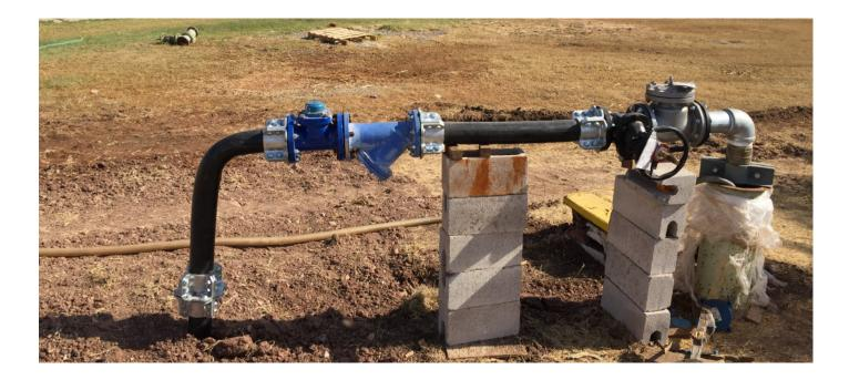
Replacement of carbon steel pipe for a Pexgol pipe
