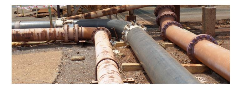
Transport of high corrosive material from the thickeners to the neutralization plant
